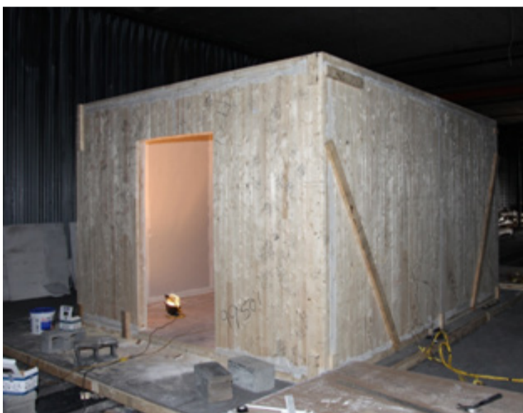
Figure 3.11. Furnished (bedroom furniture) CLT room constructed for compartment fire test conducted at Carleton University.
