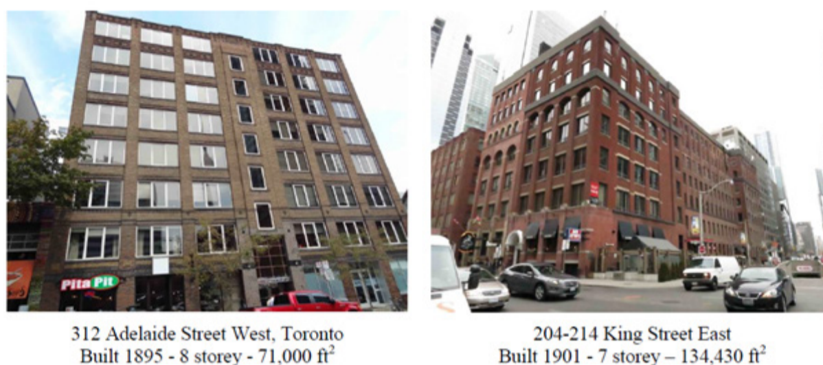
Figure 2.1. Typical brick and beam buildings in downtown Toronto. (Figure 1 from Koo, 2013).
