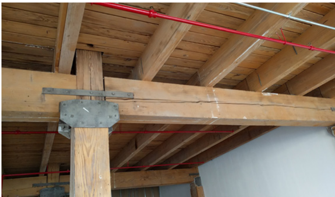
Figure 2.4 Solid Sawn heavy timber construction (Photo: A. Franco)
