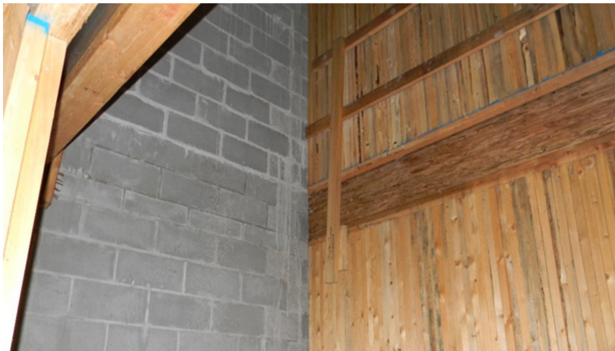
Figure 2.6 Nail-lam elevator core adjacent to masonry stair core. (Photo: M. Alexander)
