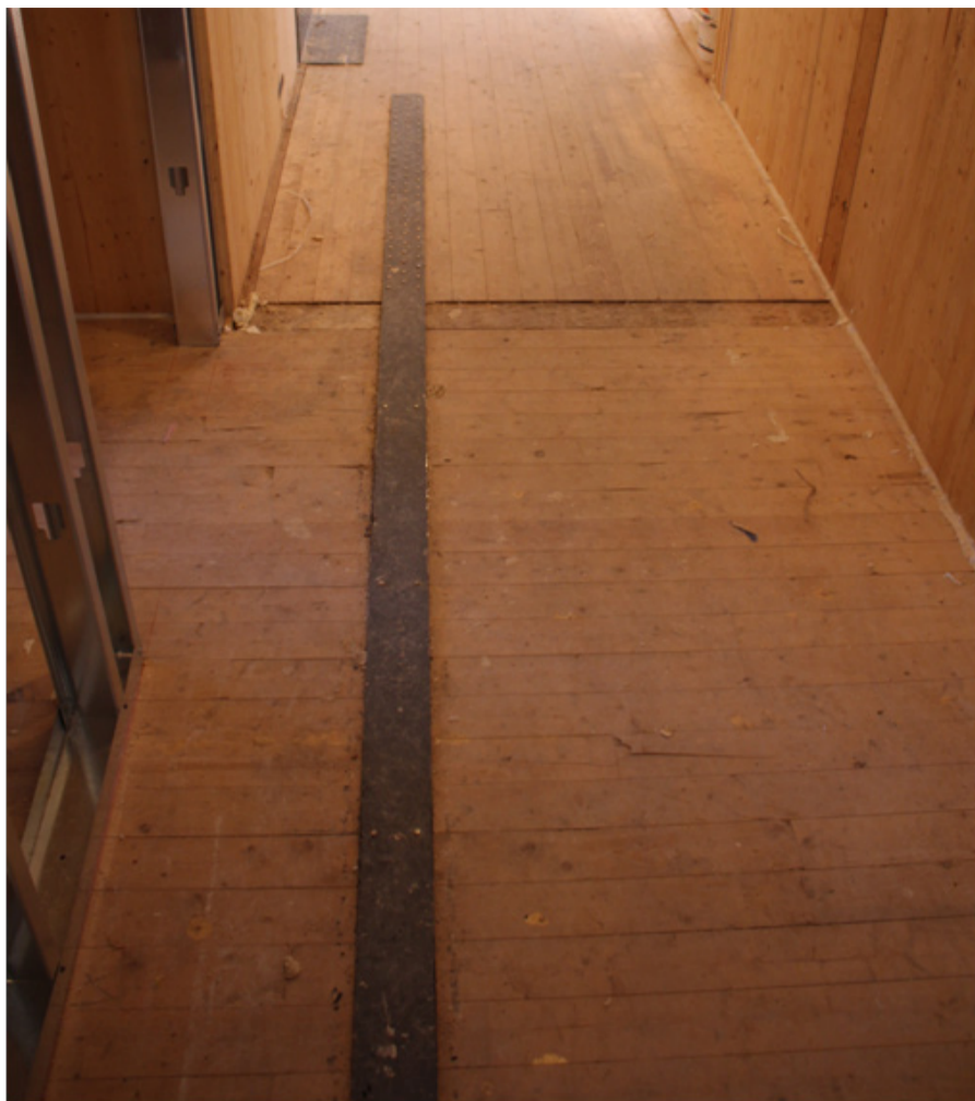
Figure 4.5. Example drag strut at Origine, Quebec city (Photo: D. Moses)
