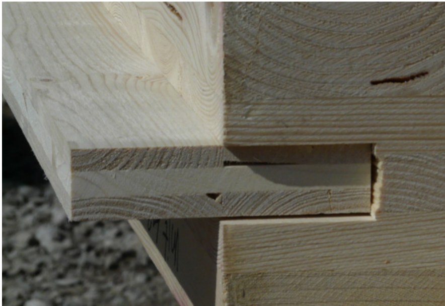
Figure 4.6. Example wall to wall panel connection (Photo: D. Moses).
