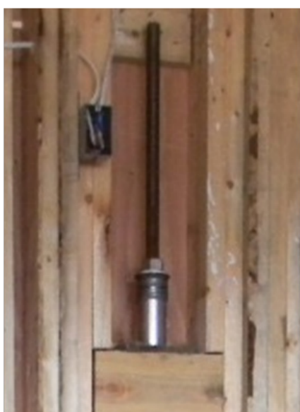
Figure 4.4. Example of a hold-down rod system with shrinkage compensator (Photo: M. Alexander)
