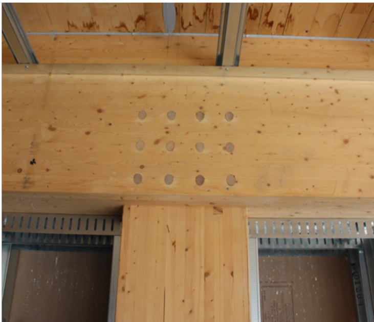
Figure 4.8. Concealed connection by Nordic, Quebec (Photo: D. Moses)
